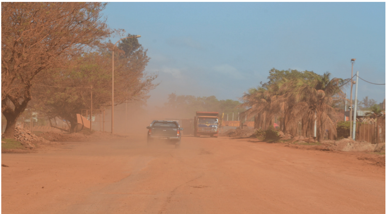
Figure 5: Road stretch toward Kuantan Port heavily covered by dark red dust
