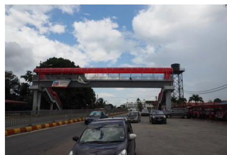
Figure 6 (b) - Pedestrian bridge far from the school gate.
