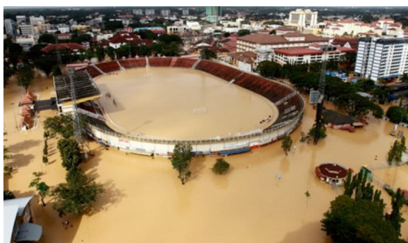
Figure 1: Kelantan Football stadium was filled with floodwaters.
